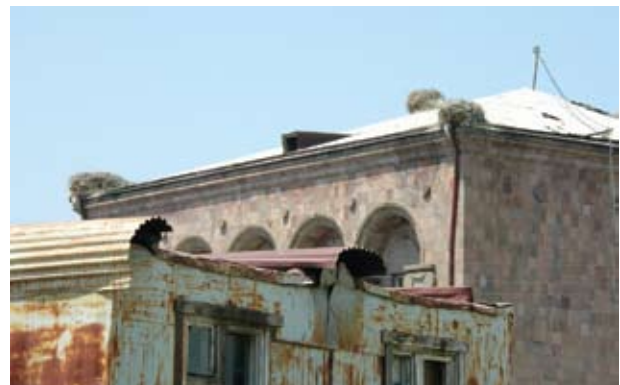
Nests on roof - Photo by Hayk Harutyunyan © Acopian Center for the Environment, AUA Nests, which block drainage pipe: the source of conflict between storks and human.
